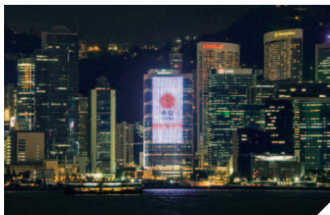
LED light decoration (35m W x 91m H) on the northern façade of CITIC Tower
