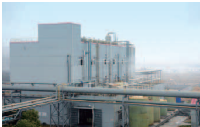
Salt extraction station for de-sulphuring effluent of Xin Yaxing Coking
