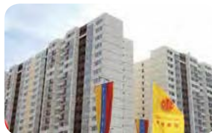
The housing handover ceremony for the D Zone of Tiuna Social Housing Project, Venezuela
