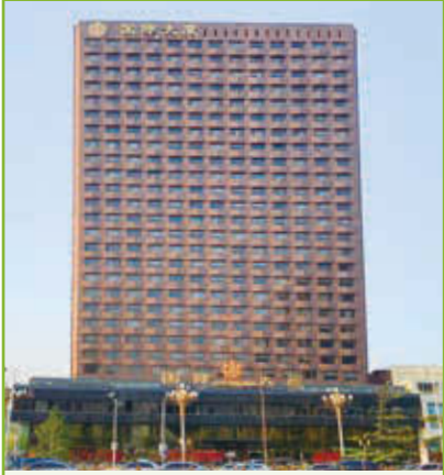
Approx. gross area: 62,200m 2 Purpose: Office
