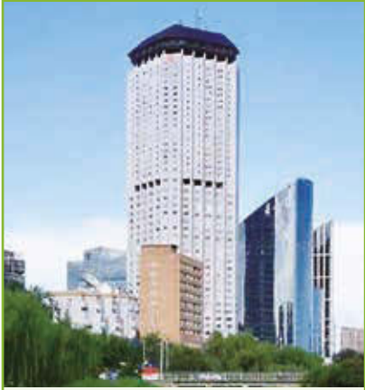
Approx. gross area: 140,200m 2 Purpose: Office
