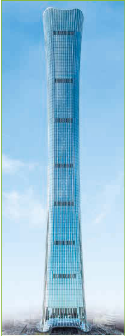
Approx. gross area: 437,000m 2 Purpose: Office
