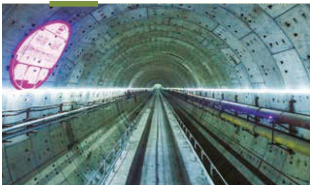
■ CITIC Urban Development and Operations opened the Shantou Bay Tunnel after successfully completing the entire project.
