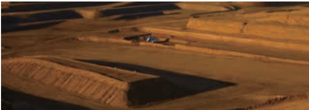
■ CBMM mine pit
