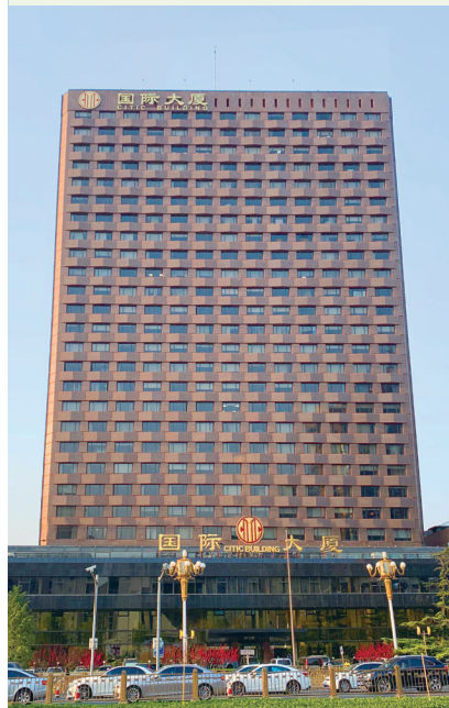
CITIC Building, Beijing (100% owned)
