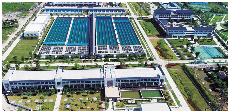
UF membrane facilities at Guangzhou, China
