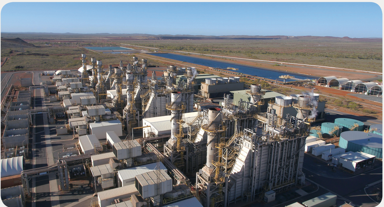
1 The Sino Iron project combined cycle power plant
