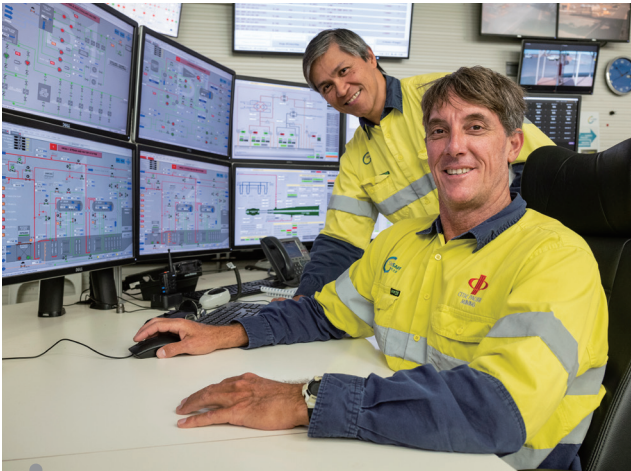
Sino Iron power station control room
