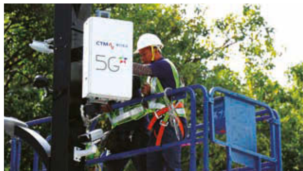
■ Installation of 5G network in Macau
