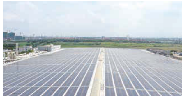
■ Sunburst's distributed photovoltaic power generation project
