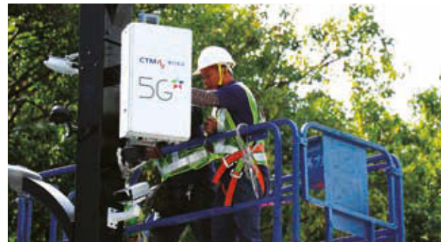
■ Installation of 5G network in Macau
