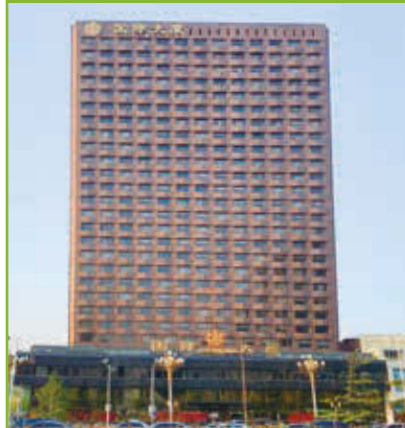
CITIC Building, Beijing (100% owned)
