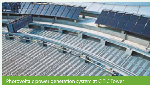
Photovoltaic power generation system at CITIC Tower
