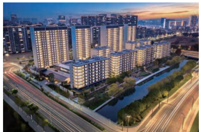
Suzhou Jiuyue Project
