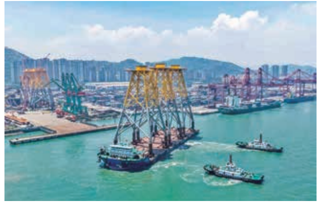
The offshore wind power jacket was shipped
