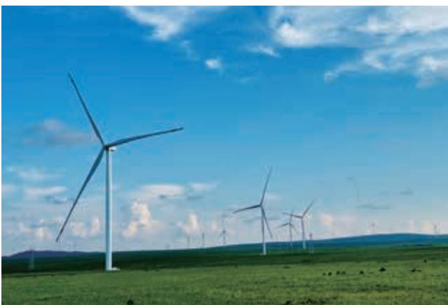
Xilinhot Wind Power Project in Inner Mongolia
