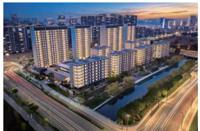
Suzhou Jiuyue Project
