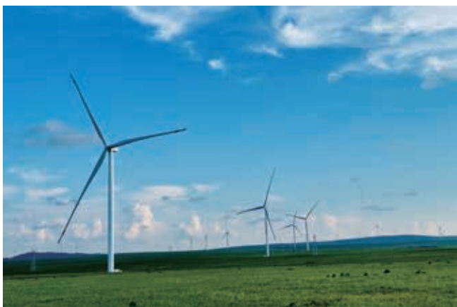
Xilinhot Wind Power Project in Inner Mongolia
