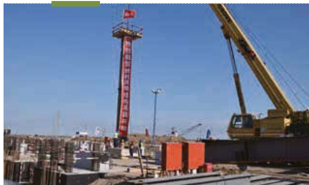
■ CITIC Construction started erecting the steel structure of the combustion engine room at Misan Power Plant in Iraq
