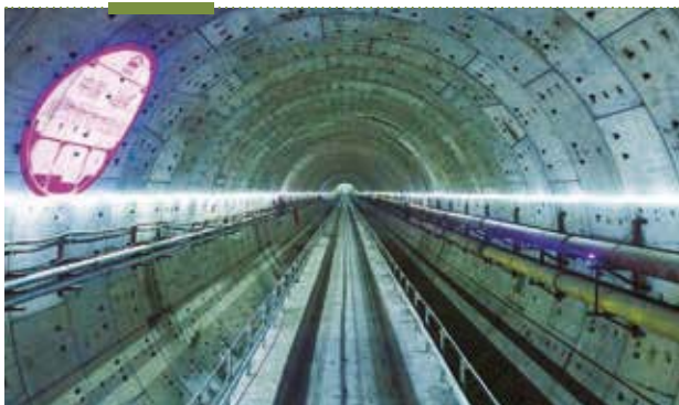
■ CITIC Urban Development and Operations opened the Shantou Bay Tunnel after successfully completing the entire project.
