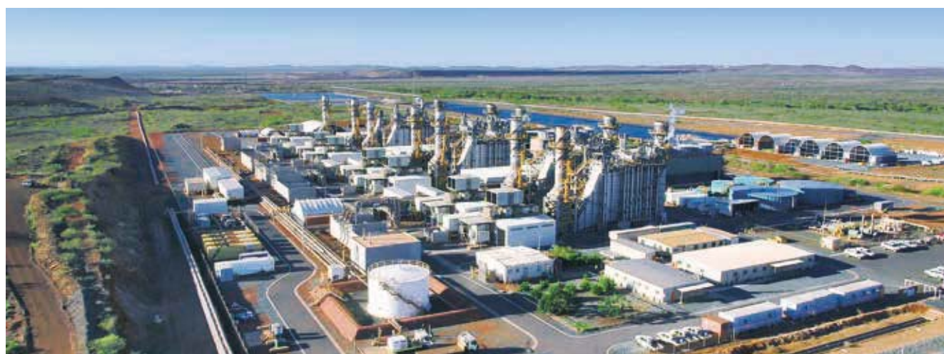
View of CITIC Mining International's energy-efficient gas combined cycle power plant
