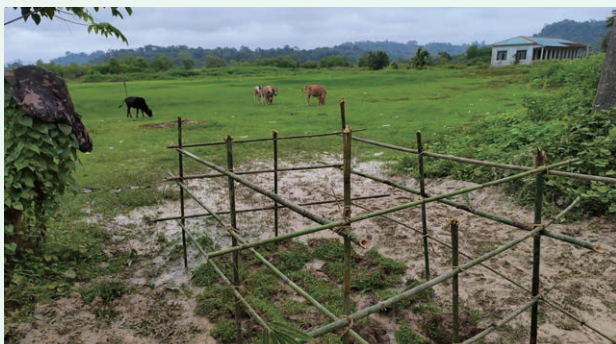
CITIC Construction carries out ecological restoration of land-based exploratory pits
