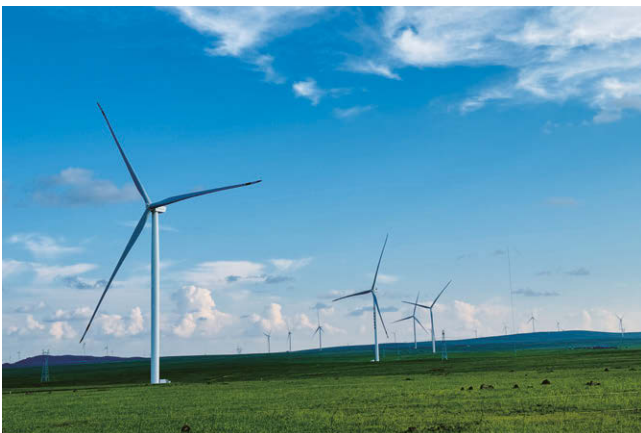
Xilinhot Wind Power Project in Inner Mongolia
